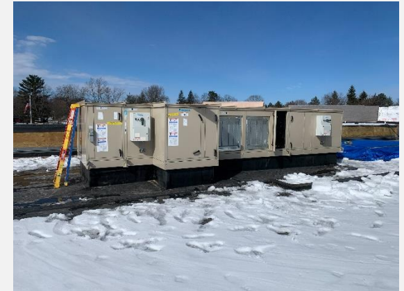
Delivery & Installation of Rooftop Units
