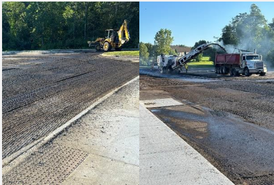
Asphalt milling and replacement paving in progress
