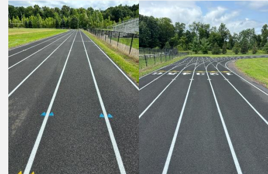
New track asphalt subbase, rubber, and striping complete
