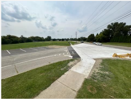
New north lot asphalt parking and concrete approach
