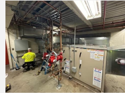
New air handling units being piped and powered in mechanical mezzanines
