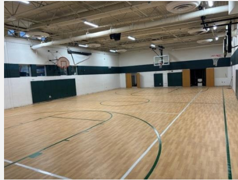
Auxiliary gym flooring replacement and striping complete
