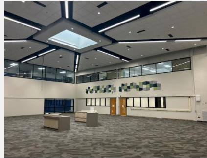
Media Center ceiling, millwork, and finishes nearing completion
