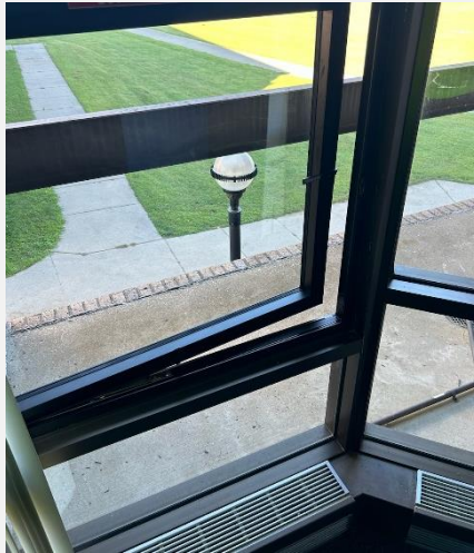
Pine Tree Center Operable Window Repair
