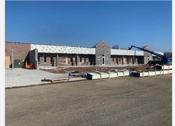
Metal Panel Installation
