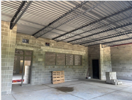
Area A addition dry-in complete.
