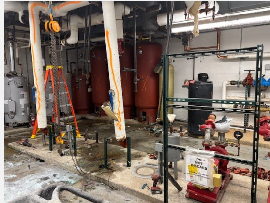
Boiler Room demolition in progress.
