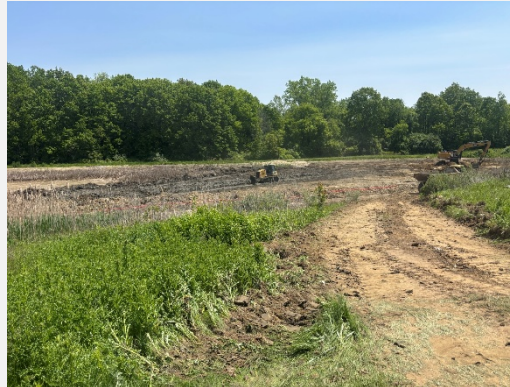
Reshaping of existing detention pond in progress.
