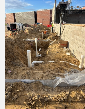
Underground utility work around new addition complete
