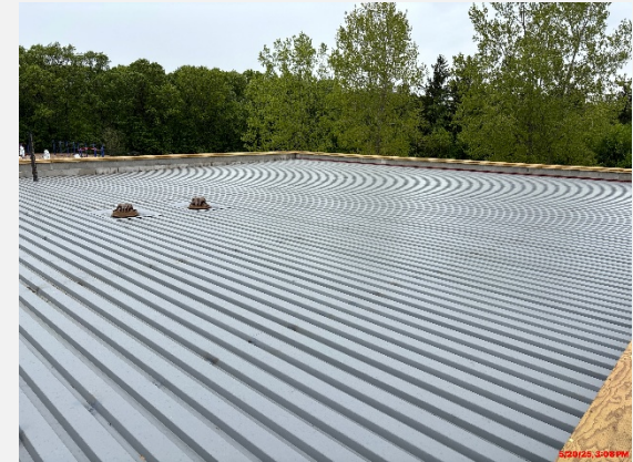
Area A roofing complete.
