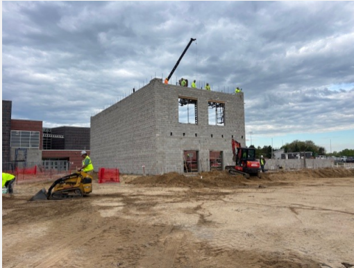
Masonry block walls in progress.
