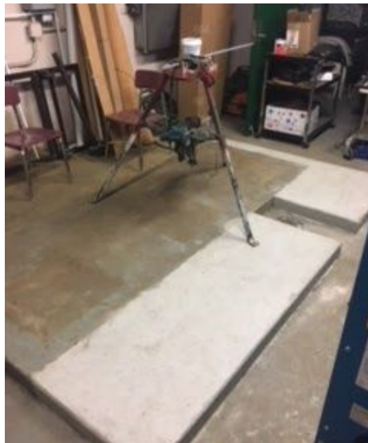
Orion Oaks- Boiler Demo and Floor Preparation.
