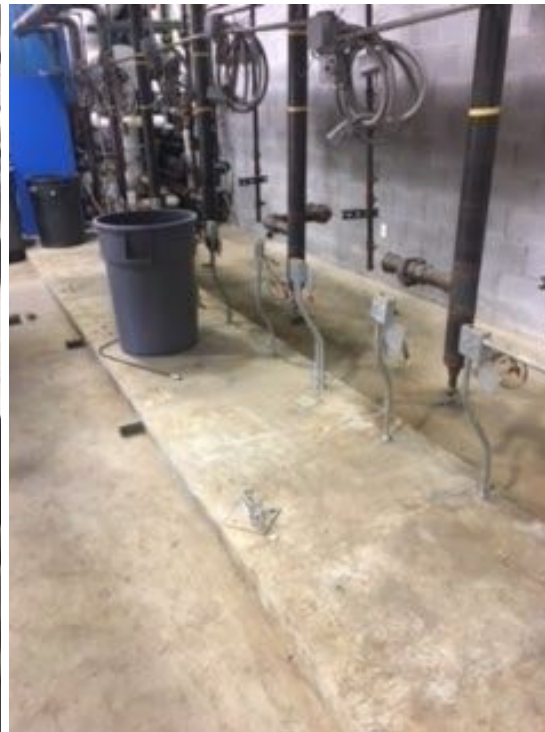
High School- Preparation for New Boilers
