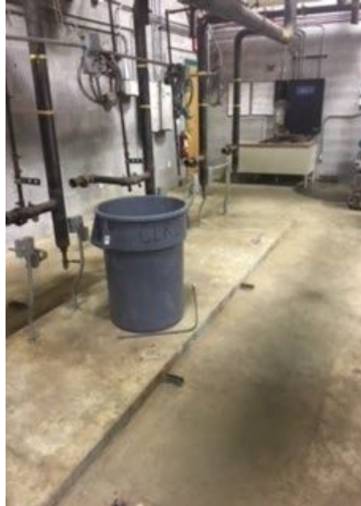
High School - Demo of Boilers
