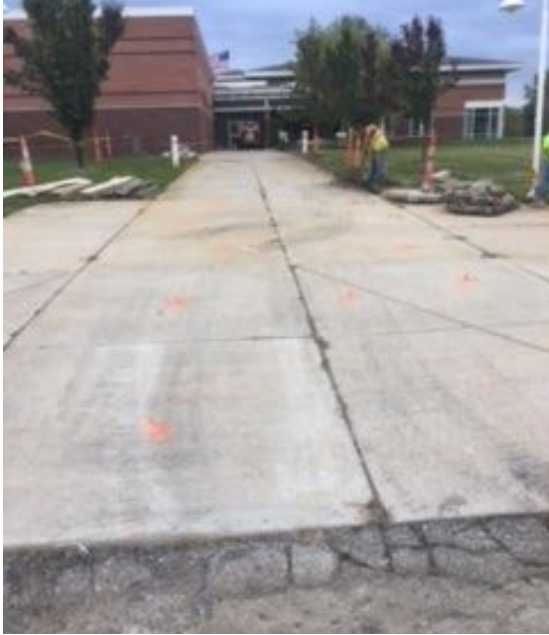
Oakview Middle School- Bus Entrance Concrete
