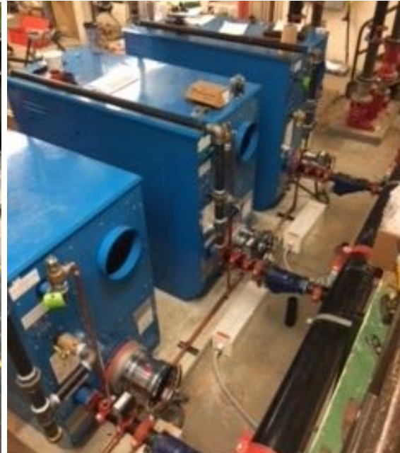
Scripps- Boiler installation
