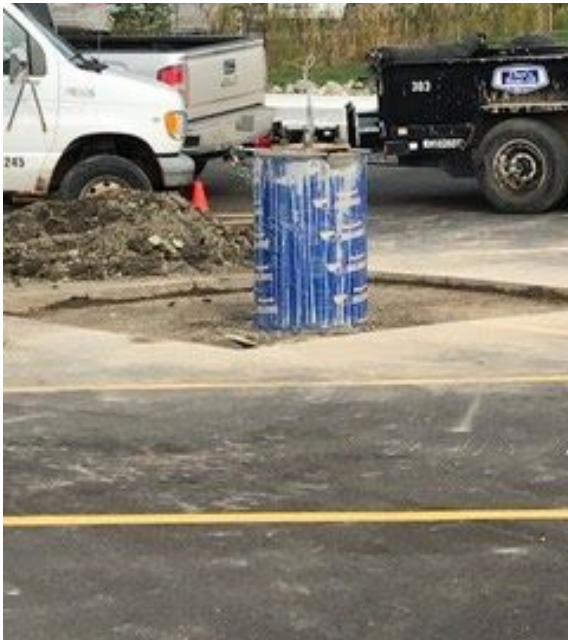
Stadium Drive Ele.- Light Pole Base Replacement
