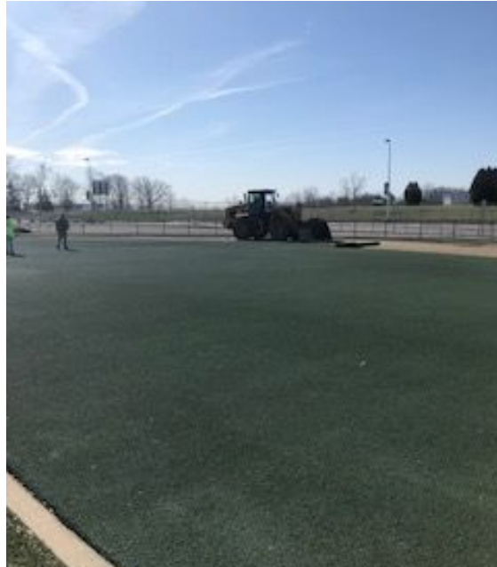
High School- Track Surface Demo
