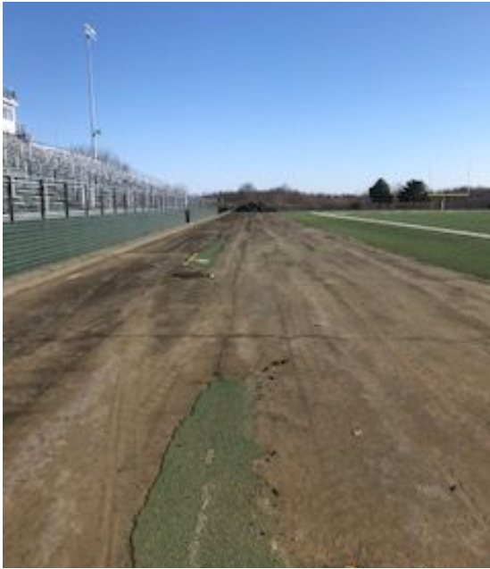
High School- Track Surface Demo
