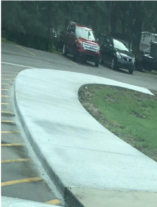
Blanche Sims- Concrete Replacement
