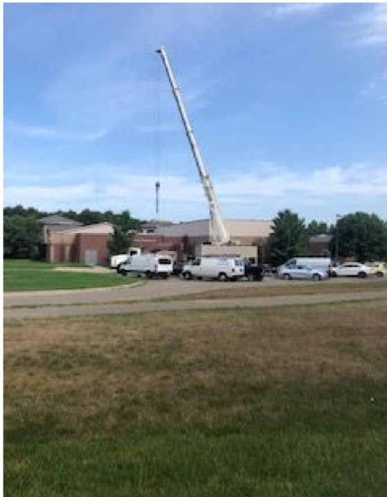
Paint Creek- Chiller Replacement
