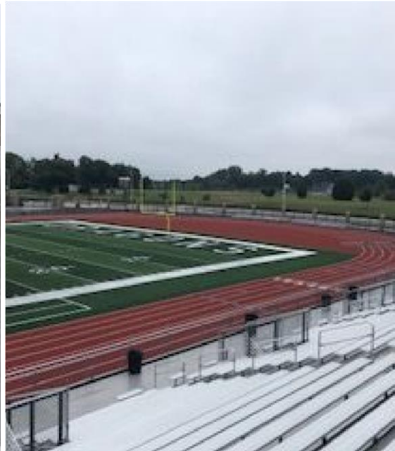
High School- Turf and Track Completion
