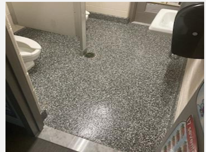
New Epoxy and Marble Thresholds in Classroom Bathrooms
